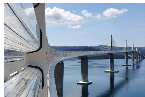
Wind Louvers Gap
