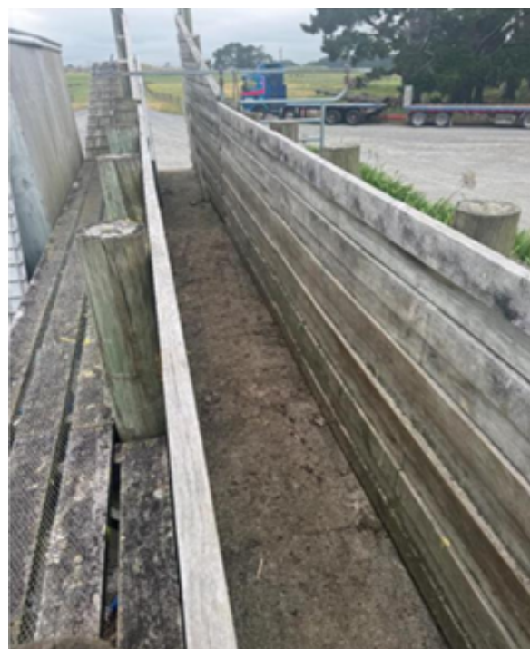
Figure 5. Loading race with catwalk access to the crate door
